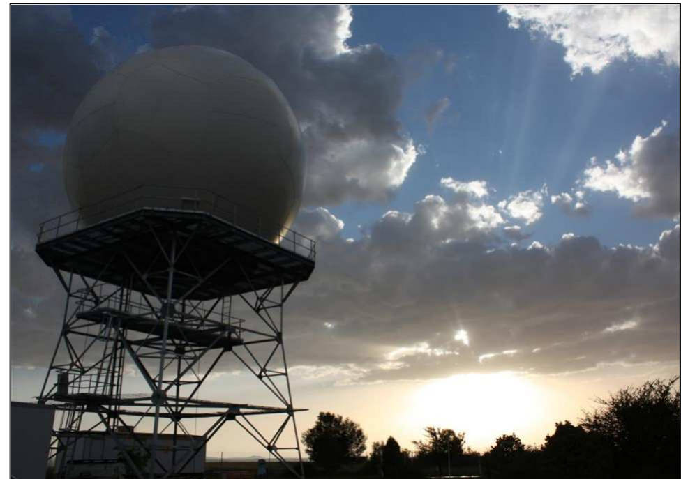
S-Band installation in Bethlehem
